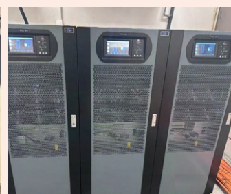
The upgraded centralised UPS (left) and its battery (right) at Menara OCBC.
