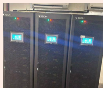
The upgraded centralised UPS (left) and its battery (right) at Menara OCBC.
